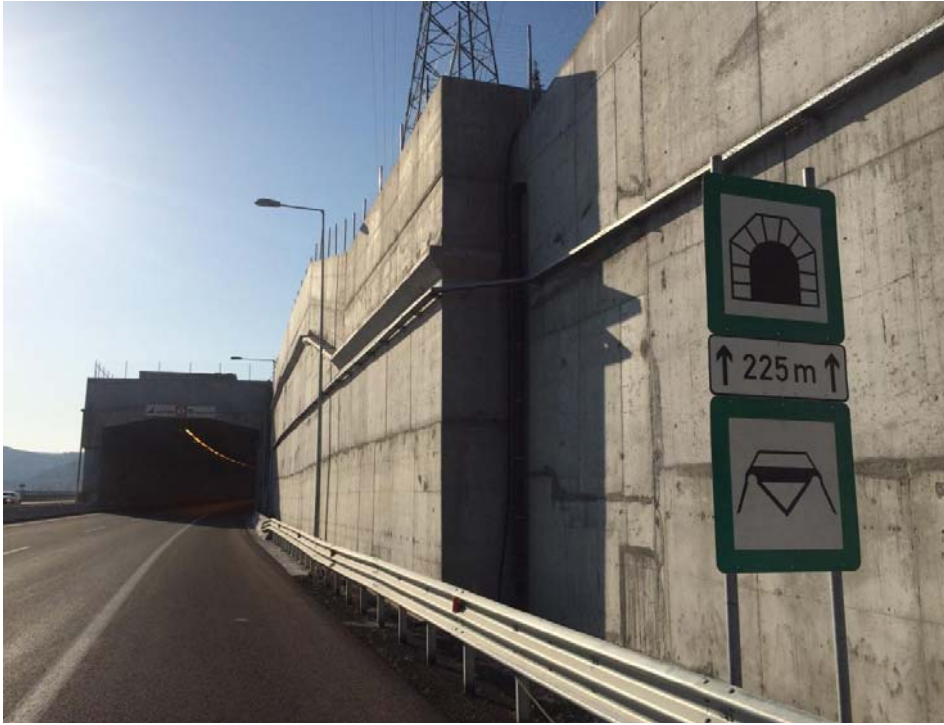
Fencing at side roads
