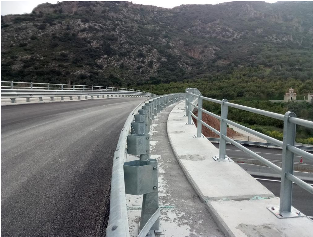
A223 – Replacement of safety barriers and placement of safety guardrails
