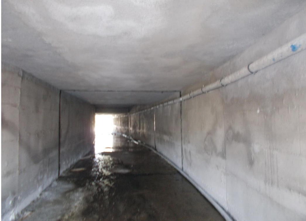
Rehabilitation works at culvert S050
