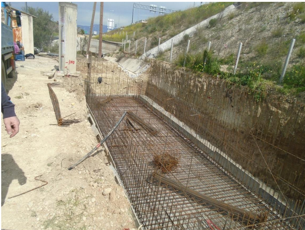
B131 – Construction of decantation tank
